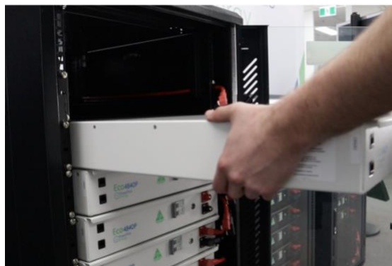
Figure 8 – Typical Battery Assembling
