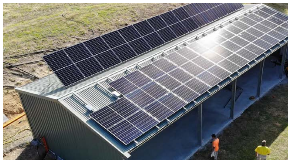
Photos courtesy of JPM Electrical and Solar (March 2021)
